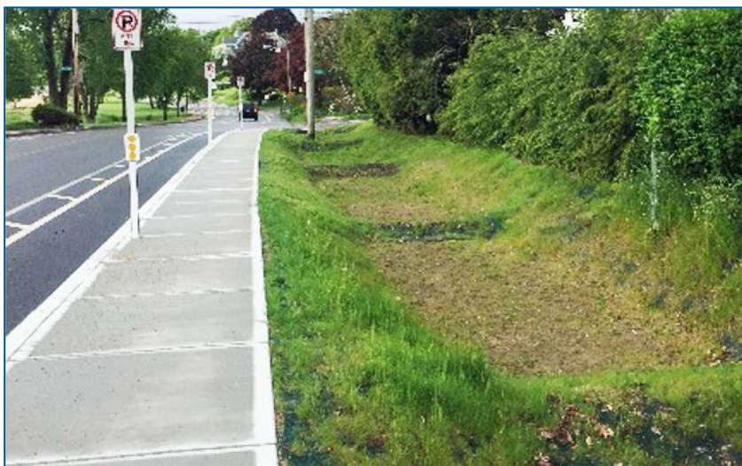
Bioretention Swale in Cranston, RI. Photo courtesy of Fuss and O’Neill, Inc.
